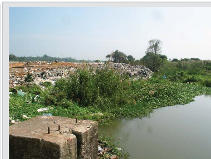
Figure 1. Unplanned garbage dumping area in the BAS. Credit: D.M.S.S. Karunarathna
